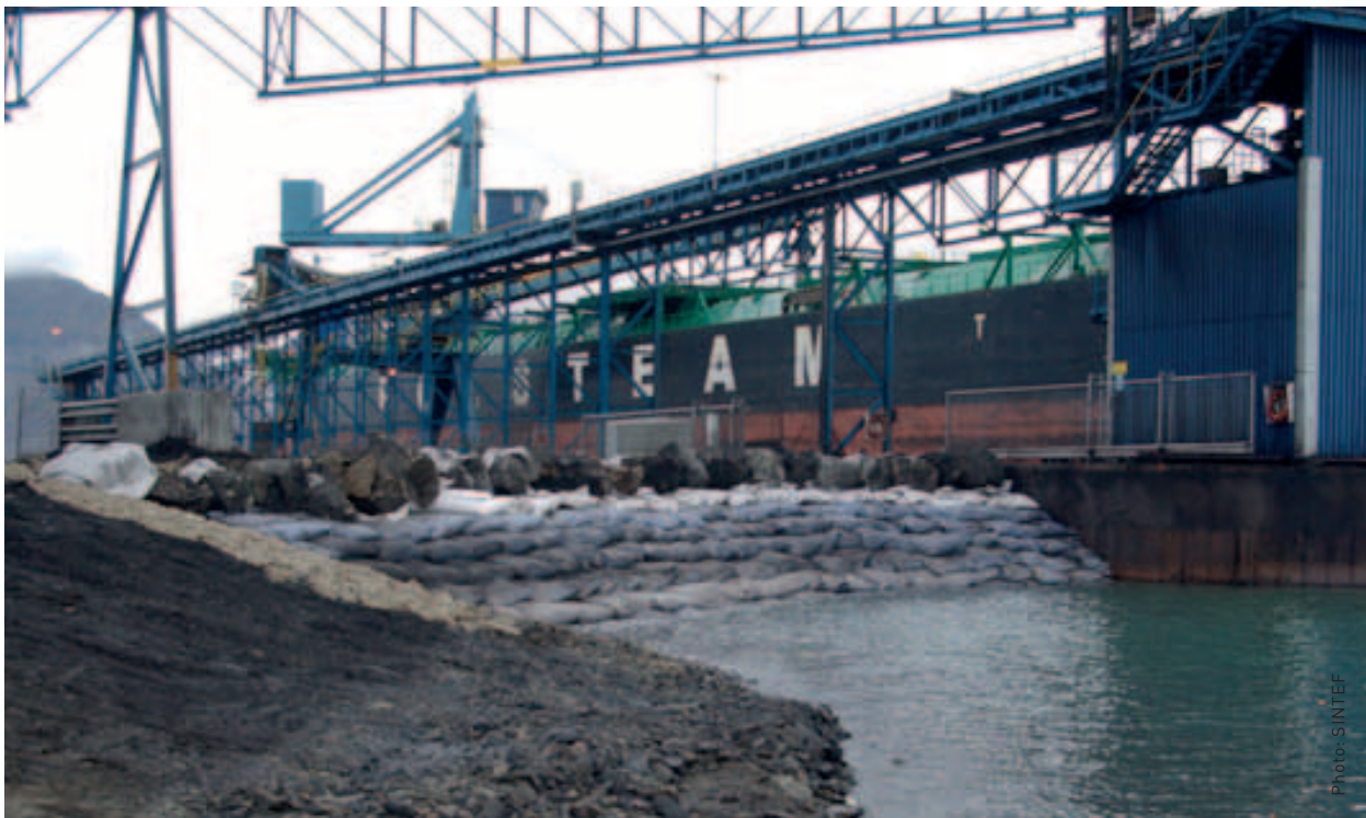
Erosion protection in Kapp Amsterdam, Svea.
