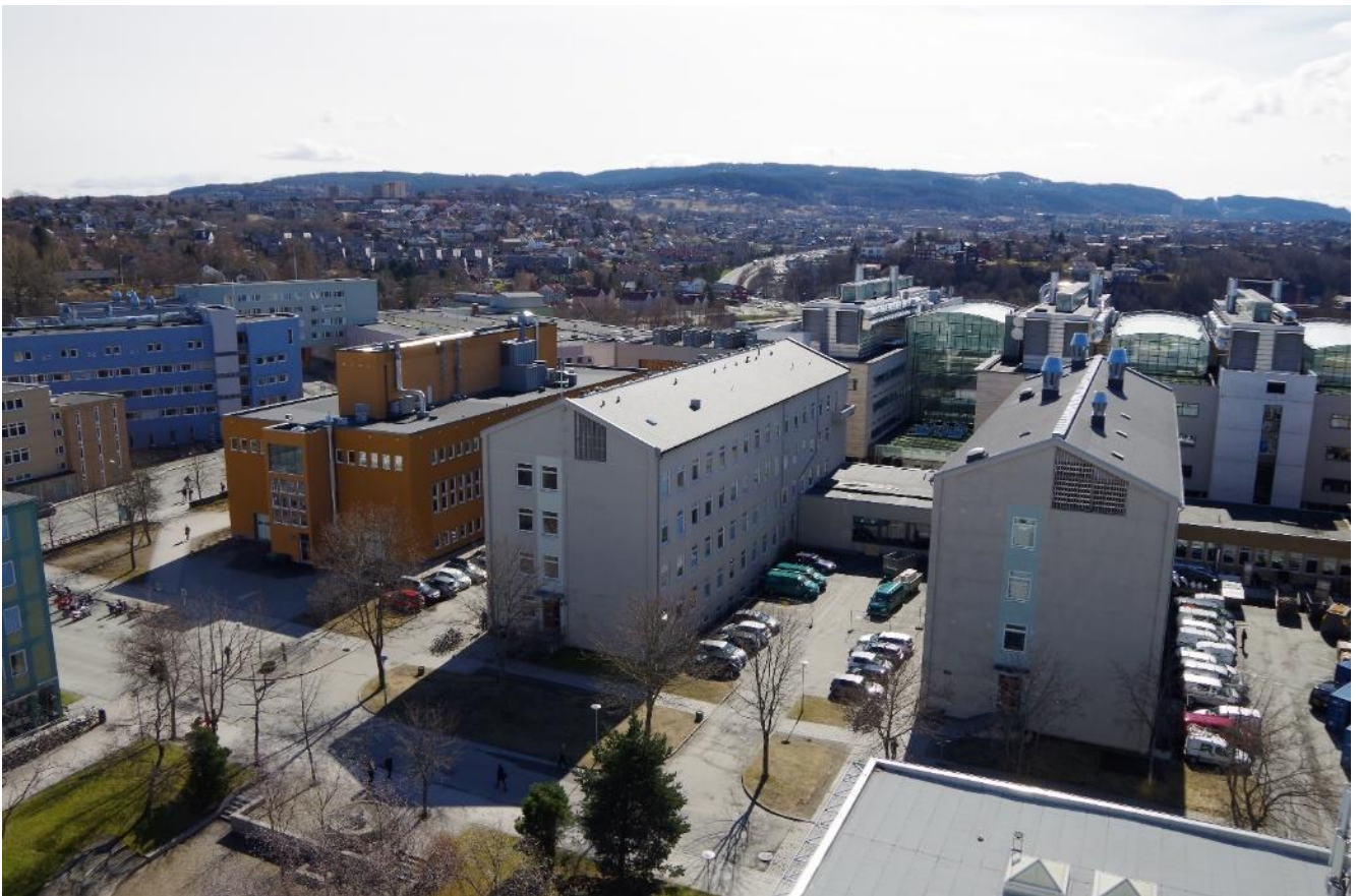
Our buildings, from the right: K4, K5, Experimental halls and the PFI-building (blue)
