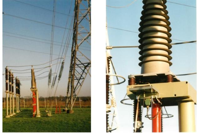
Figure 3. 150 kV substation with two parallel circuits (left) and a capacitive sensor installed next to a termination (right).
