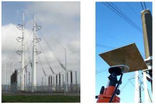
**Figure 6.** 380 kV overhead line to underground power cable transition (left) and installed sensor near a cable termination (right).
