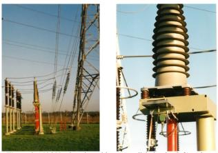
Figure 3. 150 kV substation with two parallel circuits (left) and a capacitive sensor installed next to a termination (right).
