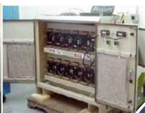
Source: Electricity Storage Association, 2009.
