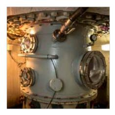
Plexiglass windows are installed on the draft tube of Svorka power plant (25 MW), operated by Statkraft
