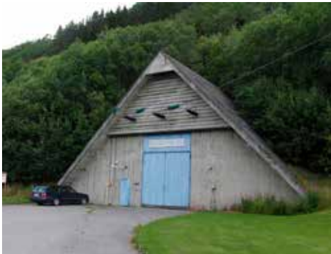
Entrance to Ylja power plant
