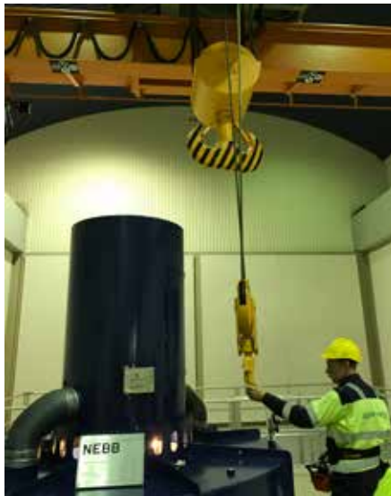
A crane used as a fixed reference to demonstrate the vibrations during a visit in October 2017
