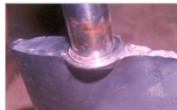
Erosion in GV of Jhimruk HP, Nepal.
