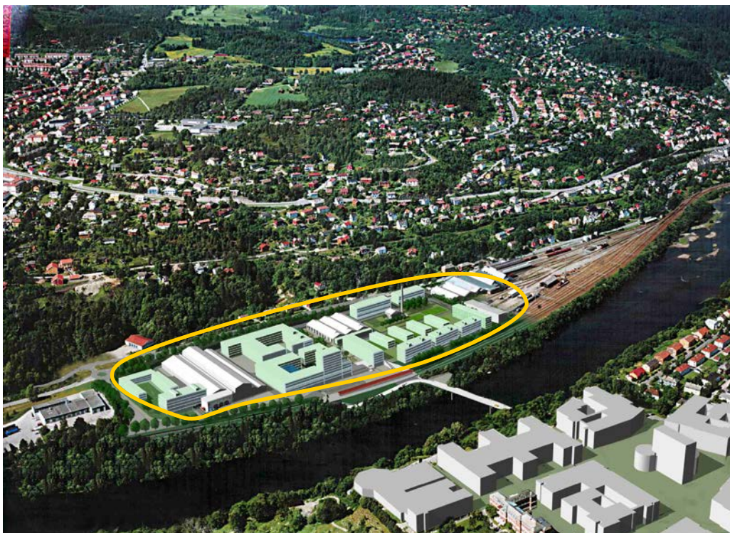
Figure 1. Illustration of the approved plan of Marienborg. The railway on one side and the road on the other side of the site give good access. A large hospital development is under construction on the other side of the river.
