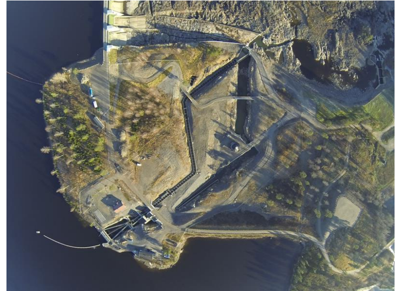
Fish ladder at the Stornorrfor powerplant in the Ume river.
