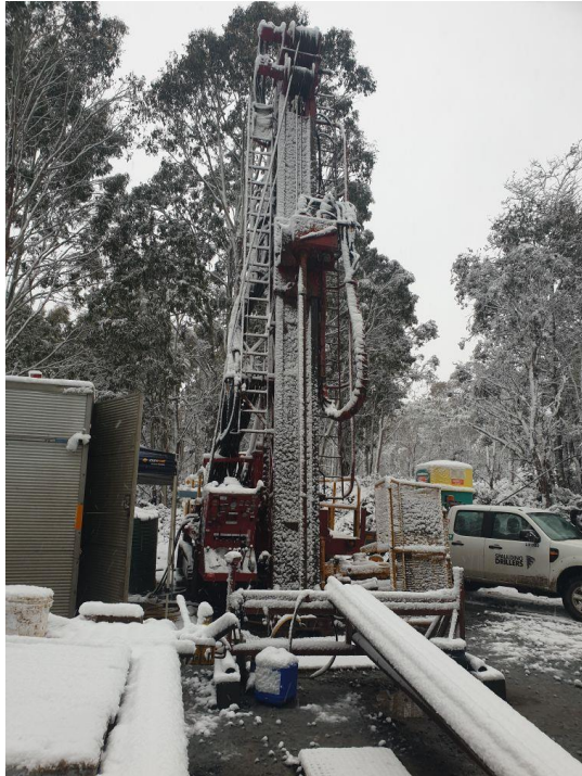
Photos of geotechnical drilling underway at Lake Cethana PHES site
