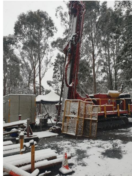
Photos of geotechnical drilling underway at Lake Cethana PHES site
