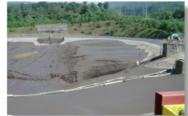
Peaking pond at El Canada HPP
