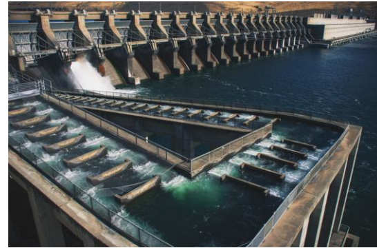
Fish ladder at John Day Lock and Dam, U.S. Army Corps of Engineers
