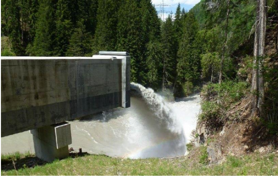
Sediment bypass tunnel outlet at Solis HEPP Switzerland
