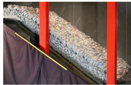
Placed riprap without toe support
