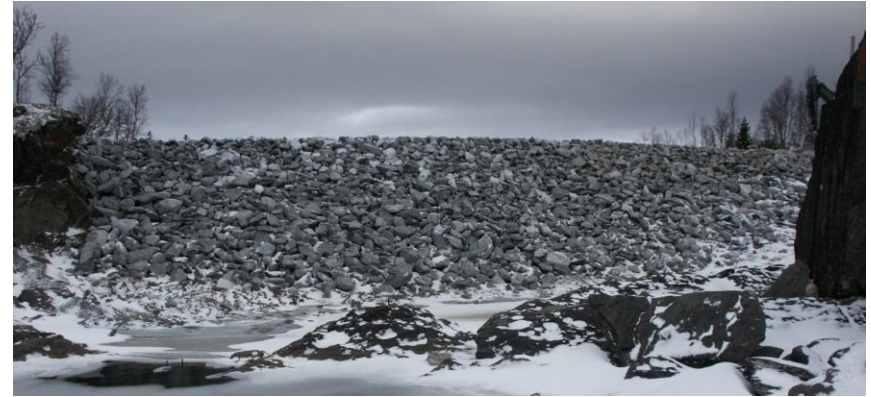
(6 m high test dam at Rossvatn, Norway)
