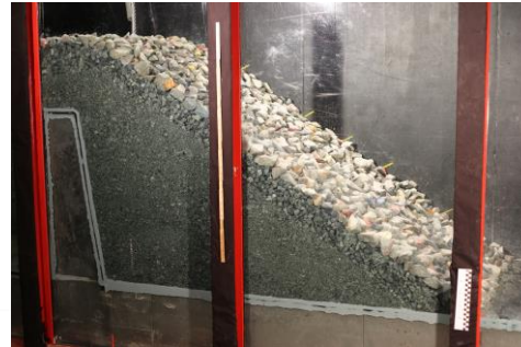
Rockfill dam with dumped riprap
