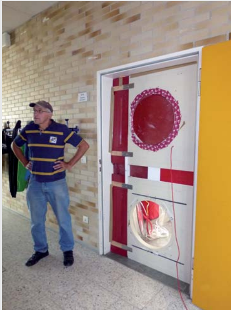
Airtightness test at the Solitude-Gymnasium
