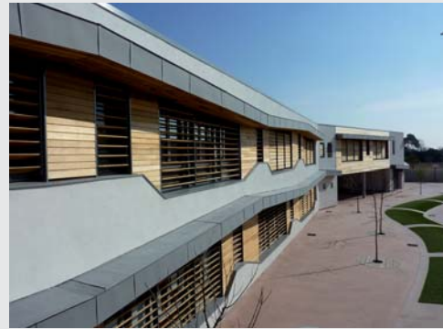
Energy surplus school 'François Mitterrand' in Montpellier
