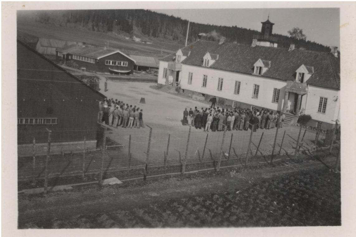
Figure 1: Picture probably taken in 1945 of the eastern Prisoners barrack and main building. Photographer: Erling Nordholmen. From the archives of the Falstad Centre. Archive number 0800311.
