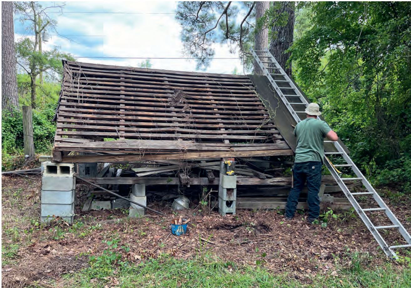
Figure 5. My brother removing nails from the roofing tin to reveal closely spaced runners that once held shingles. Photo: Christopher Witmore
