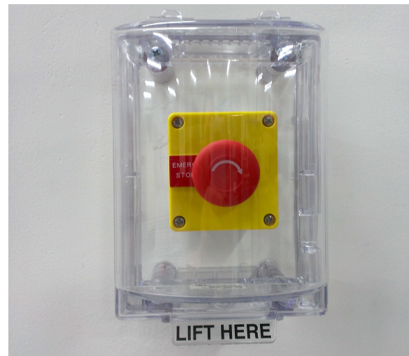
Figure 4: A retrofitted safeguard for an emergency stop button (Wahl, 2013).
