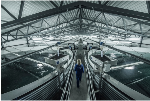
Figure 1: Land-based indoor facility using tank solution as the aquaculture structure. Sisomar AS aquaculture plant, Norway. (Photo by AKVA group, 2018)
