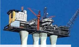
By 2007, there were 34 concrete platforms installed in the North Sea. The Troll platform (1995) is the largest. It stands in a water depth of more than 300 m. With a total height of 472 m, this concrete structure is higher than the Eiffel Tower, and holds the record as the largest structure ever moved by humans.
