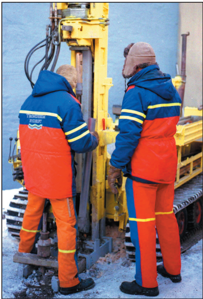
Figure 33 Use of track-mounted mechanical auger for creation of water sampler boreholes (E. E. Peacock).
