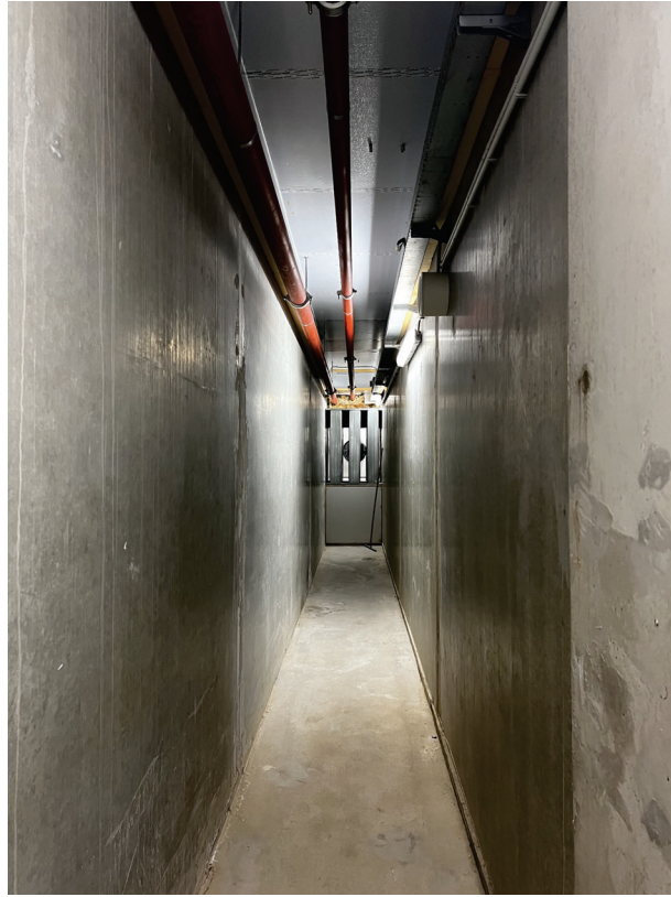
Figure 4.2.9: The walls of the labyrinth heat or cool the ventilation air, Photo taken by the author.
