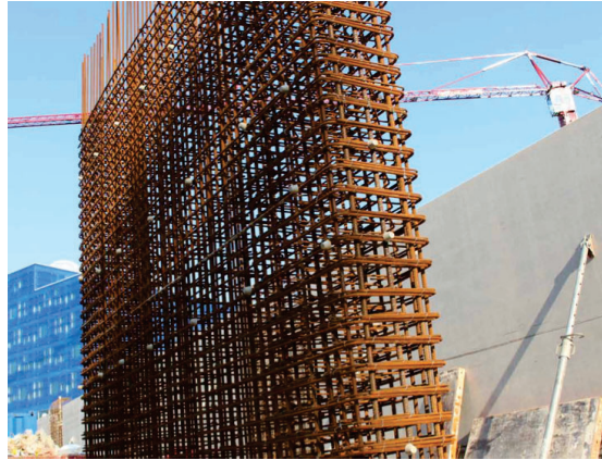
Figure 4.2.15: Six seismic walls are in place to absorb possible earthquakes( Energy Academy Europe , 2017).
