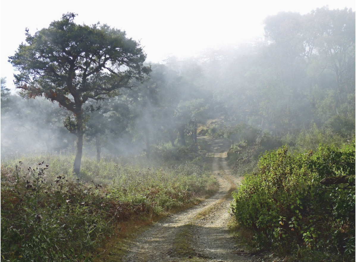
Figure 6. The Kanpetlet – Mindat road goes through the park; the upper pictures show the new construction work and the preparation for the significant extended road by felling the edging forest. This widening of the road represents a severe encroachment in the landscape, in particularly as long as the current road hurls itself with much more gentleness up and down the hills (lower picture). Photo: Per Gustav Thingstad
