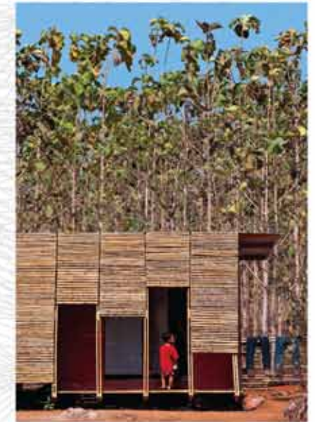
TYN tegnestue. Student project in Thailand 2009. (Photo: Pasi Aalto)
